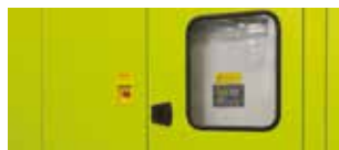
Control panel doors (one each side)
