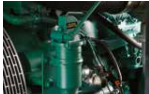
Lube oil drain pump
