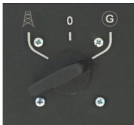
Main/generator selector switch
