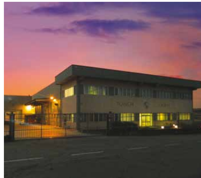
TOWER LIGHT FACTORY - ITALY
